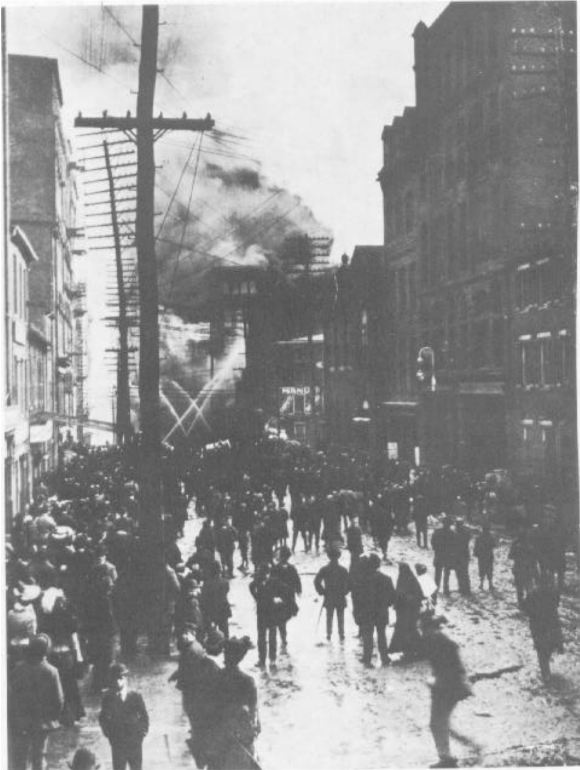
Major turn-of-the-century fires, such as Baltimore's in 1904, aroused concern about fire safety in buildings.
